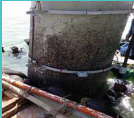
BSS Tech engineers executing the CP system for Jetty at Mundra Site
