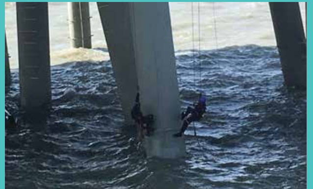
BSS Tech engineers executing the CP system for Jetty at Mundra Site
